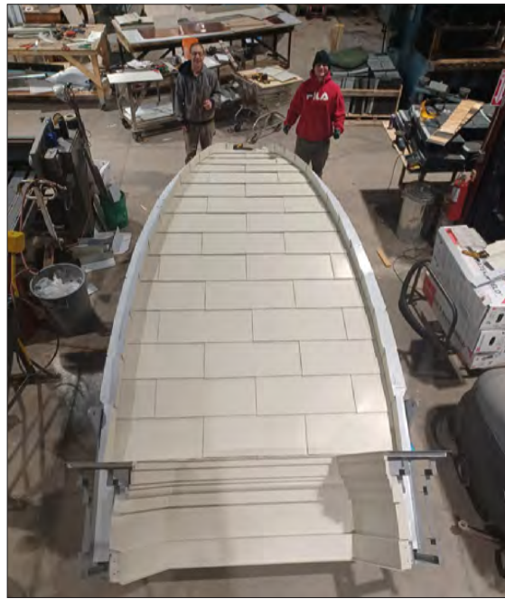
(Above) The Mason County Courthouse upper dome consisted of eight pieces which were constructed at the H&L shop in Markham, ON. H&L also fabricated 9000 spade shingles (top right) and custom louvers (right) for the project.
